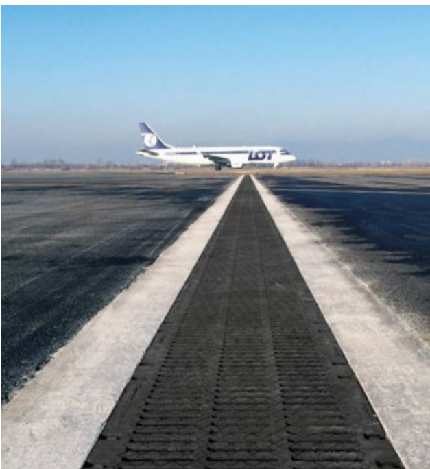
Sofia Airport, de-icing area
