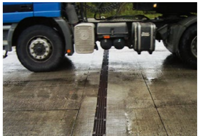
Logistics centres: Areas subject to the highest loads.
