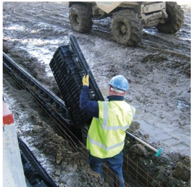
Lightweight elements, installed by one single worker.
