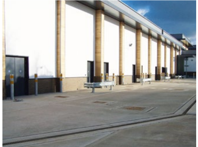
Installation in concrete surface
