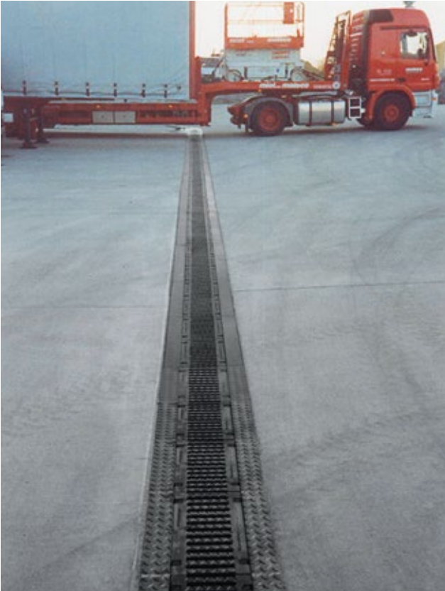
Robust and wear-resistant ductile iron protection of concrete casing
