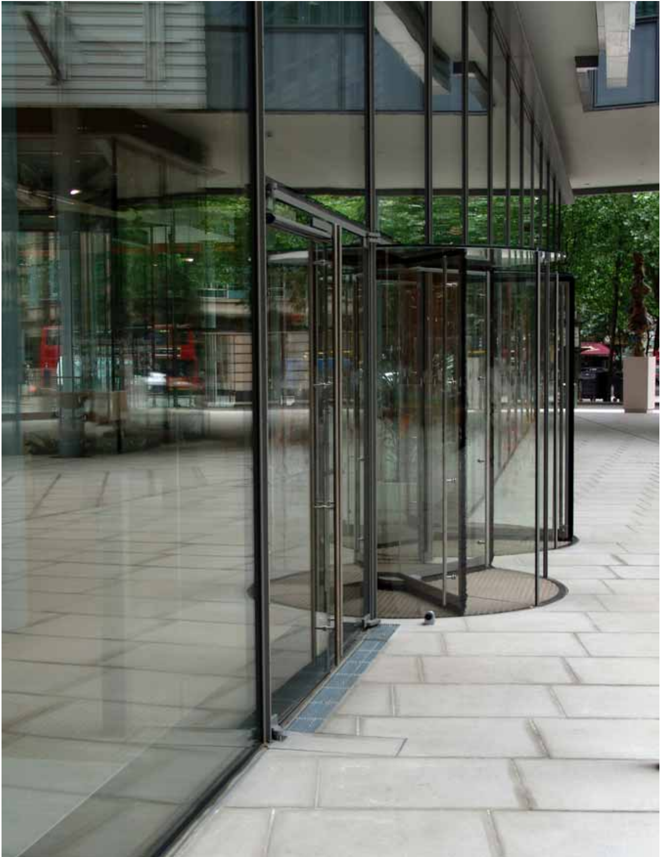
Central St Giles - BESPOKE STAINLESS STEEL CHANNELS with HEELSAFE gratings fitted at entrance doors
