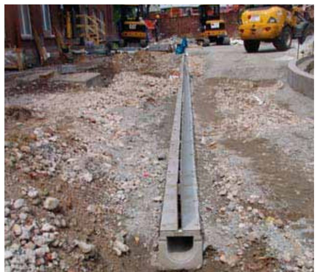
Installation of the solid Design slotted channel with grating made from 4 mm thick stainless steel and 280 mm neck height.
