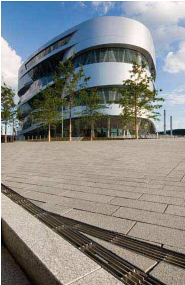
The stainless steel drainage channels were individually developed in accordance with planner specifications.
