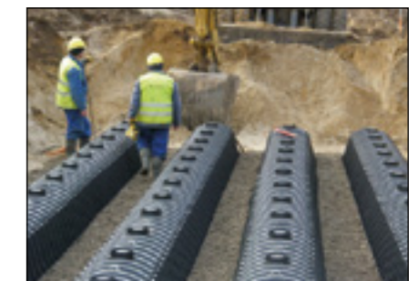
Zona industrial, Raben (PL)
