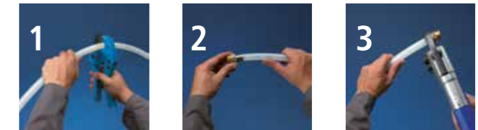
Cut the tube. Assembling accessory. Press.
