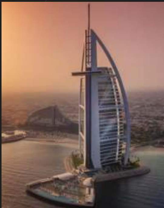
Burj al-Arab Abu Dhabi United Arab Emirates
